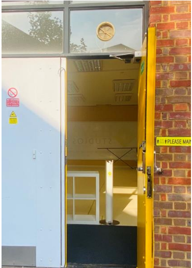
Main Door Entrance / Exit
